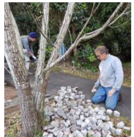
Michael O'Shea and Will Evans getting started on sorting out cobbles for new seat base
