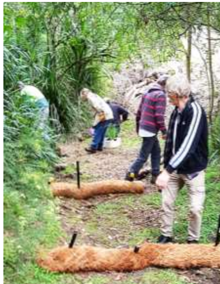
Installing sandbags at Kevin's Bridge and coir logs Grandis Gully
