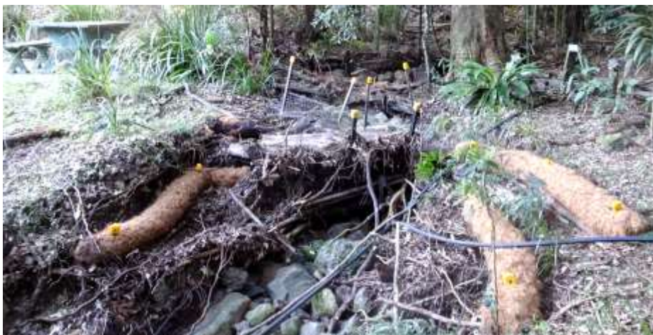
Coir logs in place in Fern Gully Creek
